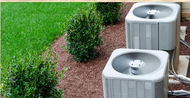
You should minimize dirt and debris near the condenser unit. Your dryer vents, falling leaves, and lawn mower are all potential sources of dirt and debris. Keep objects at least 2–3 feet away from your air conditioner on all sides to help your equipment operate efficiently. Regularly clear out any debris that gets into the coils.
